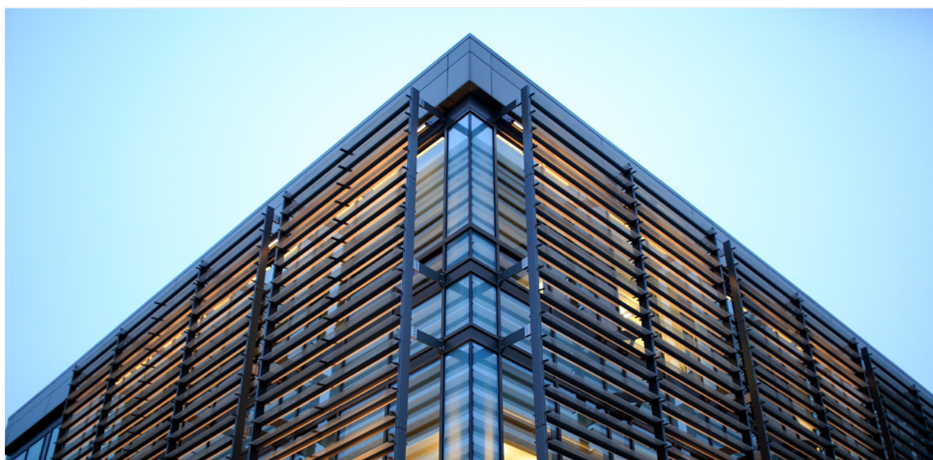
Cyberinfrastructure Building IU Bloomington Campus
